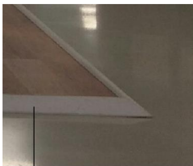
Raised floor (4cm) with sloping edges, finished with wooden laminate.
